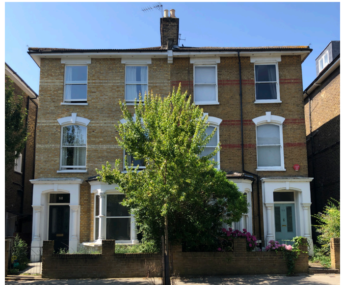
Fig 5.6 Three storey semi-detached property, Wilberforce Road
