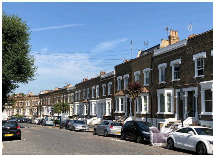
Fig 5.12 Terraced housing, Mountgrove Road
